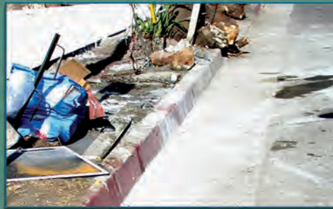
What NOT to do: Cement material dumped on a street in Santa Barbara.
