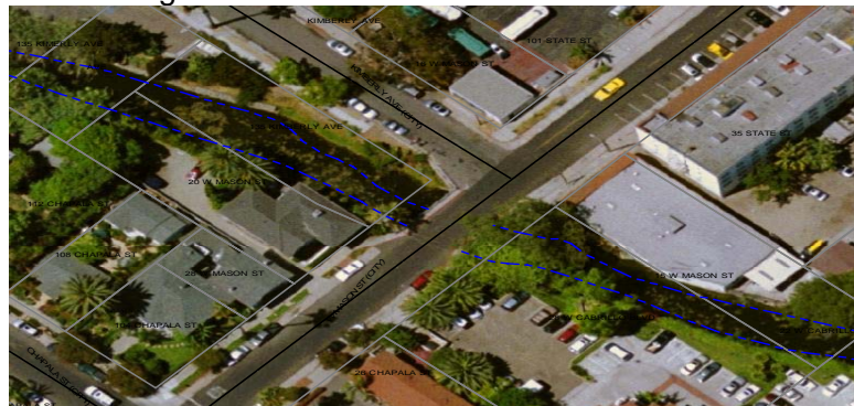
Mason Street Bridge from Aerial Photo
