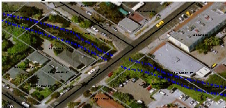
Mason Street Bridge from Aerial Photo
