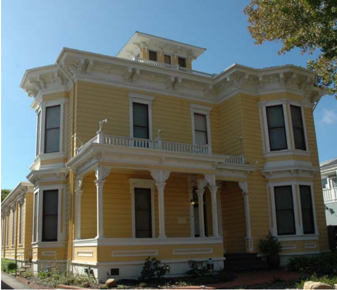
Example of a Porch
