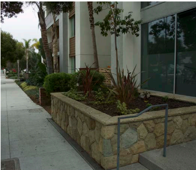
Example of raised planter on a building located near the sidewalk
