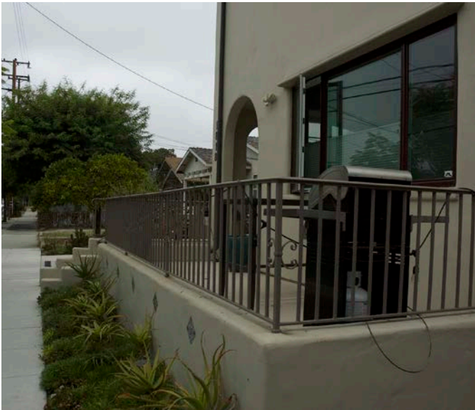
Example of a Terrace
