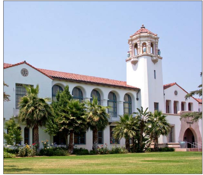
Santa Barbara Junior High School, 721 East Cota Street, 1932, (architect, William H. Weeks)
