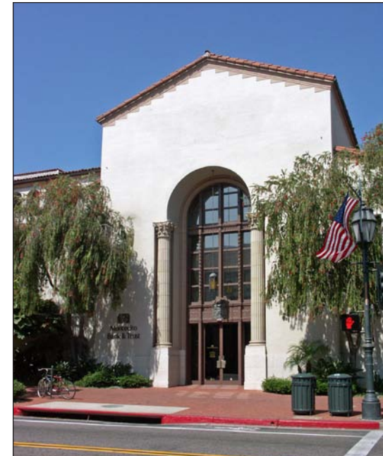
Bank of Montecito, 1000 State Street, 1921 (architect, Myron Hunt)
