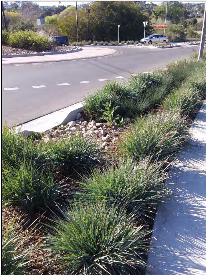
FIGURE 6-3: Roadside Swale in Santa Barbara
