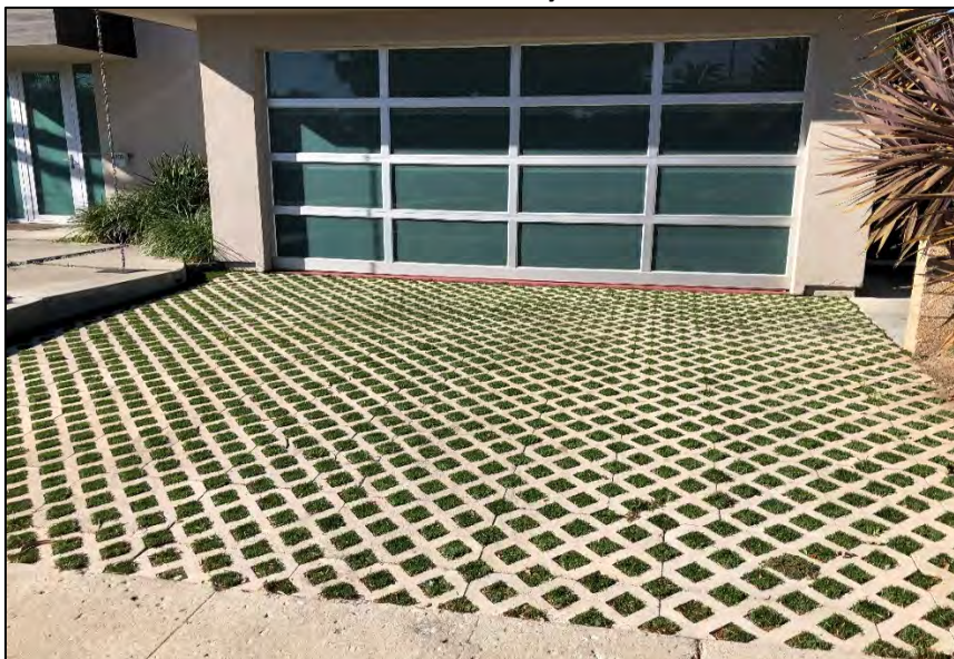
FIGURE 2-11: Grass Paver Block Driveway in Santa Barbara
