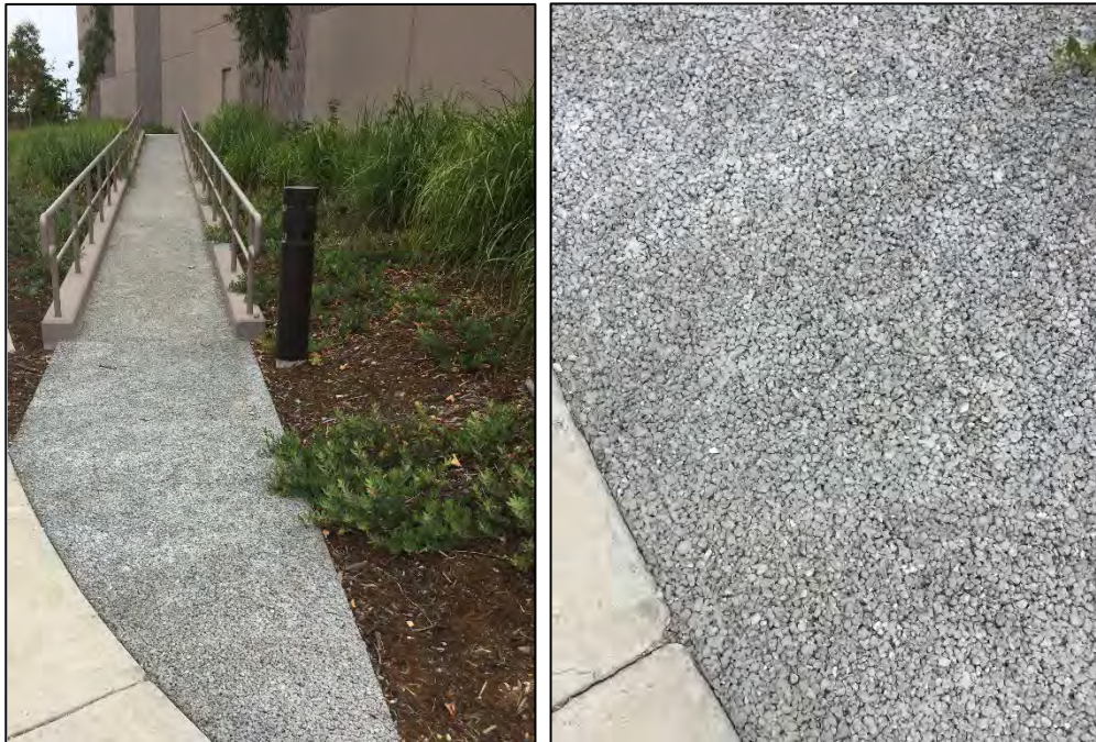
FIGURE 2-9: Permeable Concrete in Goleta
