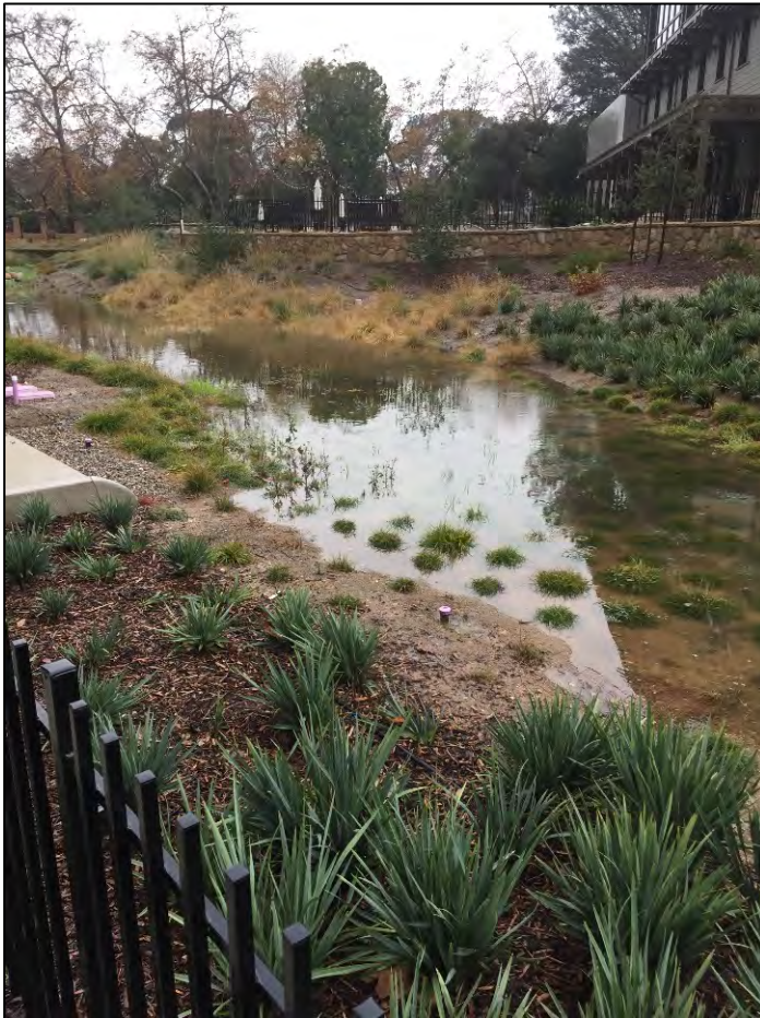
FIGURE 6-11: Infiltration Basin in Santa Barbara
