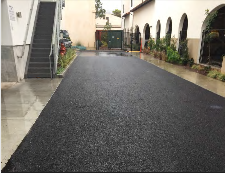
FIGURE 2-8: Permeable Asphalt in Santa Barbara
