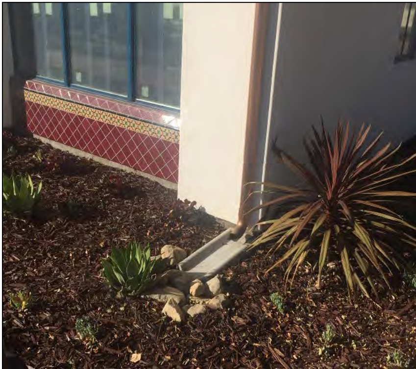
FIGURE 2-1: Disconnected Downspout in Santa Barbara
