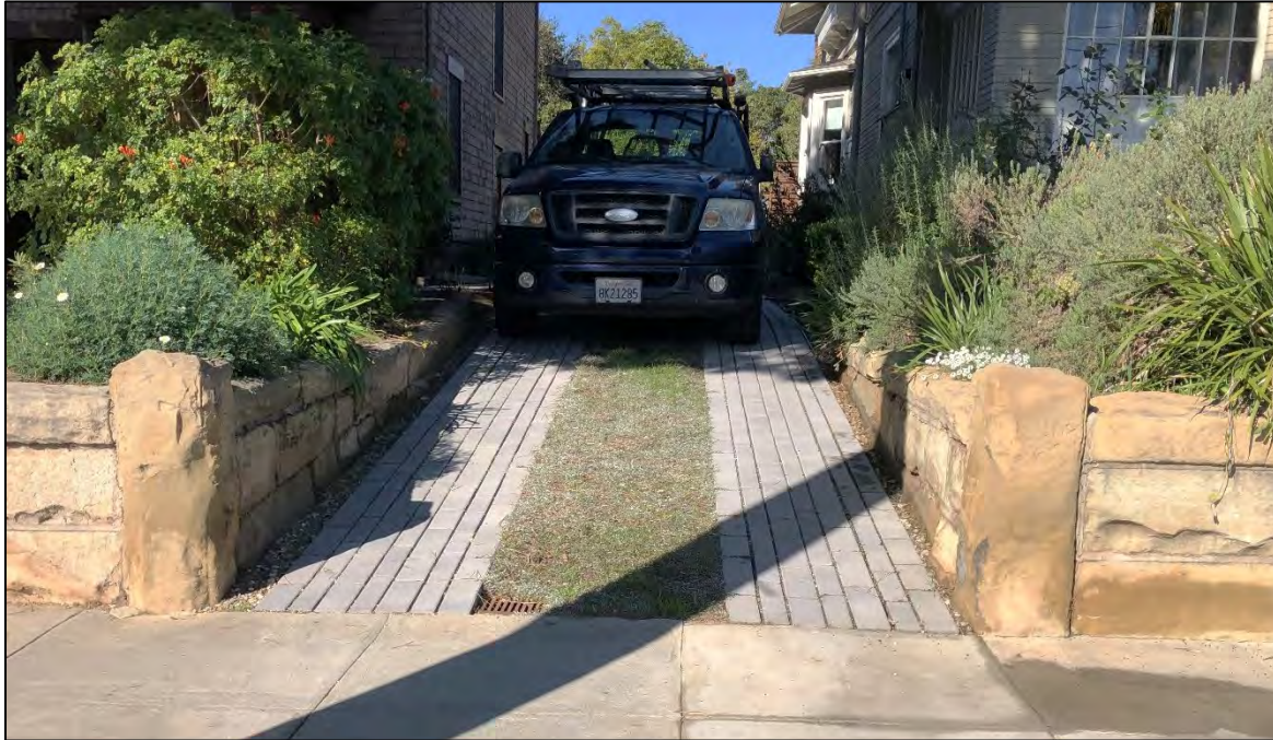
FIGURE 2-13: Ribbon Driveway in Santa Barbara
