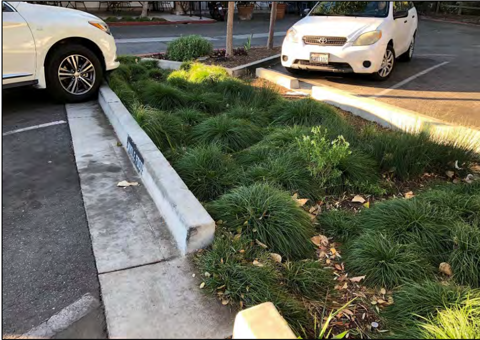
FIGURE 5-1: Example of Minimizing Impervious Surfaces in a Parking Lot in Santa Barbara
