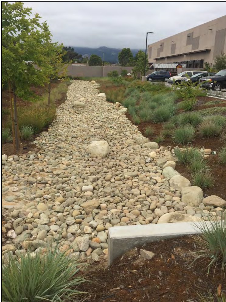
FIGURE 6-27: Dry Extended Detention Basin in Goleta
