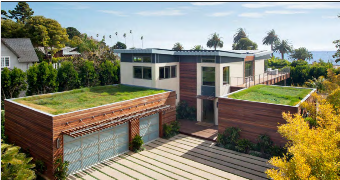
FIGURE 6-21: Green Roof in Montecito
