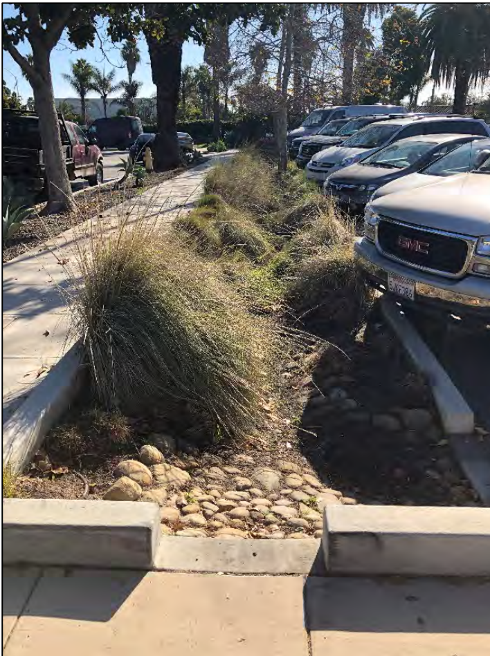
FIGURE 5-2: Example of Minimizing Impervious Surfaces in a Parking Lot in Santa Barbara
