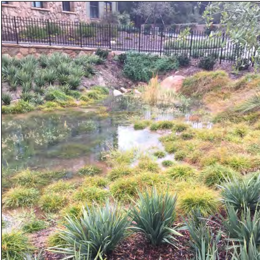
FIGURE 6-21: Constructed Treatment Wetland at 540 W. Pueblo Street
