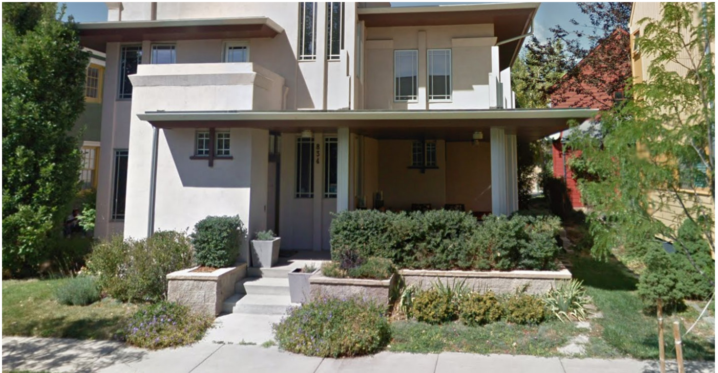
Example of a Recessed Porch (Courtesy of Google Maps)
