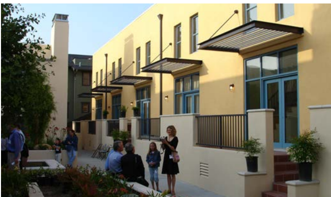
Example of a Terrace
